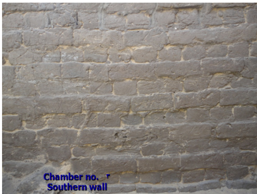
Plate 5. Details of southern wall of chamber no. 3.
