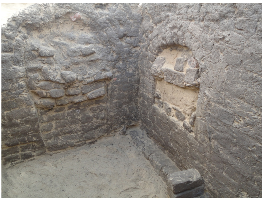
Plate 4. The eastern and southern walls of chamber no. 2.
